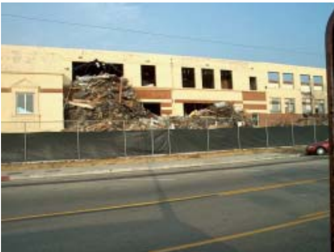
More demolition of Burbank High.
